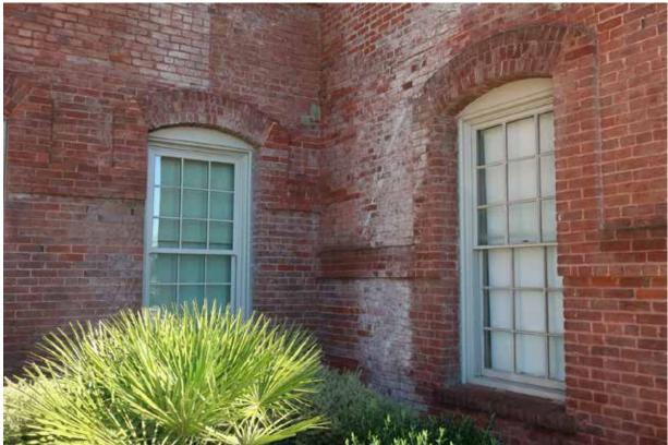
Fig.15: Petaluma Silk Mill – 2018 window at Main Building, at left; 1892 window at west tower, atright
